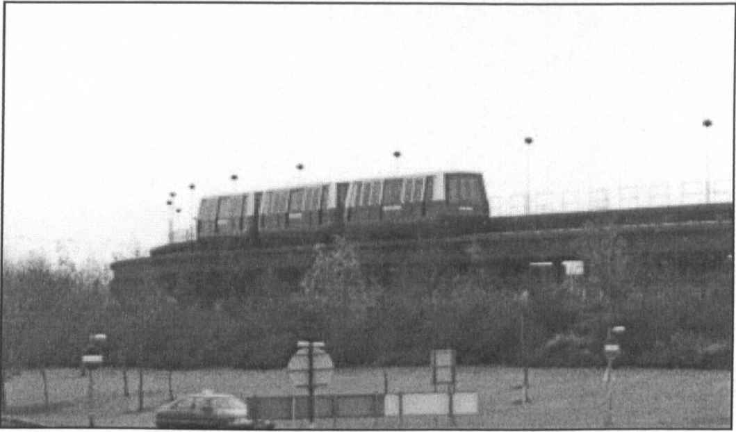
Figure 7.5 Gatwick Airport light rail 'people mover'.
