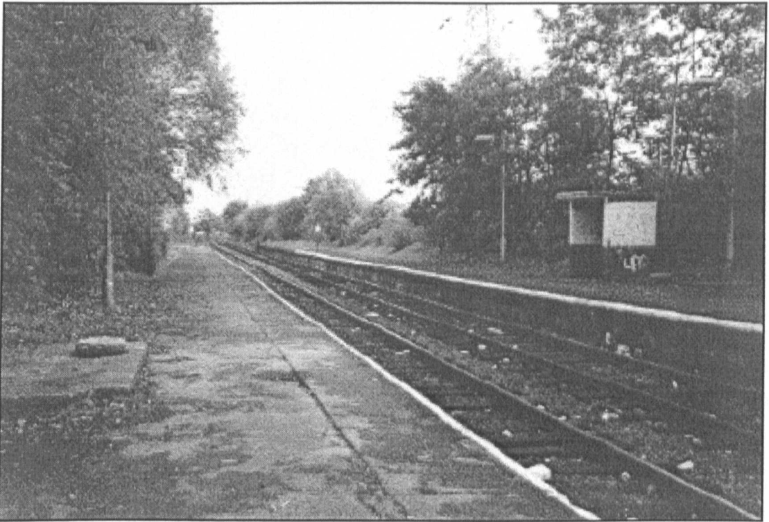
Figure 10.3 Derelict condition of Upton station, 1997.
