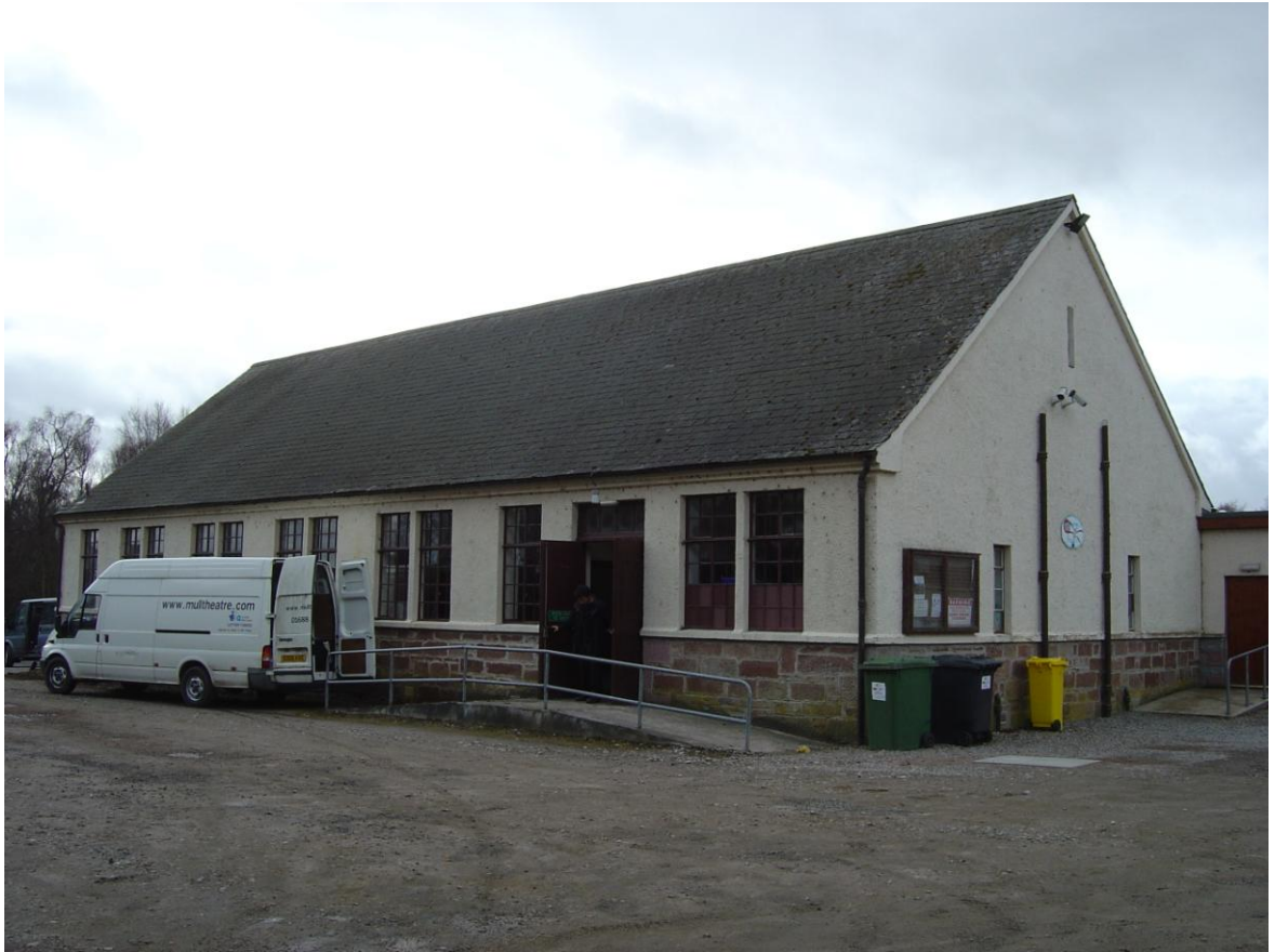
Figure 30 - Resolis Memorial Hall, side entrance
