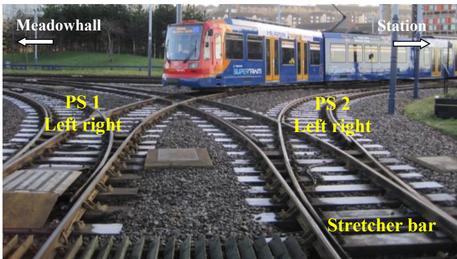
Figure 13. Configuration of the instrumented switchblades and stretcher bar on the Delta. The photograph was taken looking from the city bridge. “Meadowhall” and “Station” are significant stations on the network, and are included to allow the direction of travel of the crossing tram to be distinguished. “PS1 Left”, “PS1 Right”, “PS2 Left” and “PS2 Right” are used to identify the switch blades in the text. .
