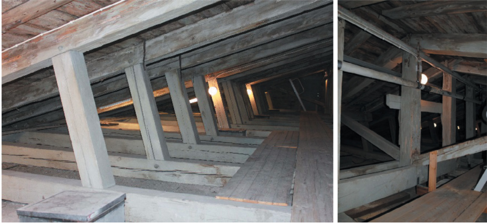
Figure 4: The roof structure no. 2.
