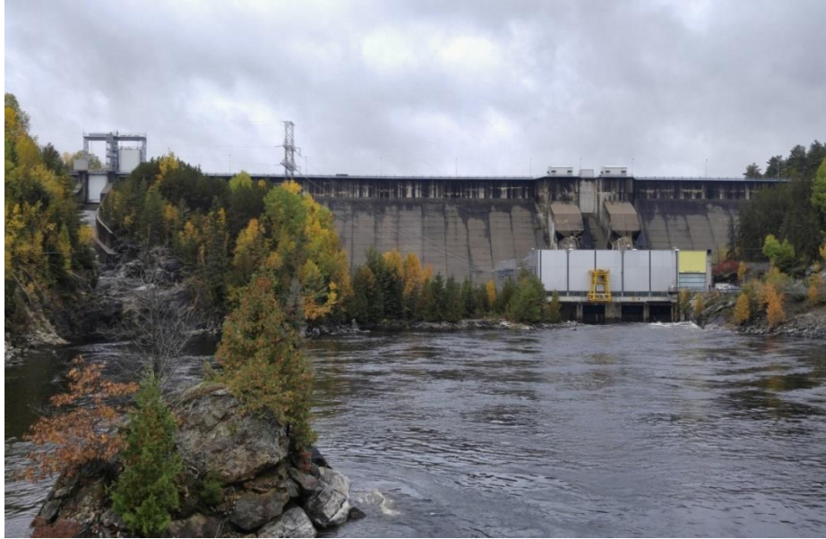
Fig.87: Mountain Chute Dam and Generating Station (sluiceway and sluice gates to the left)
