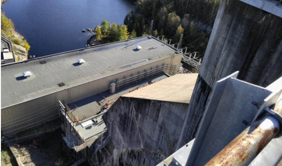
Fig.39: Penstock and Power House of Mountain Chute Dam
