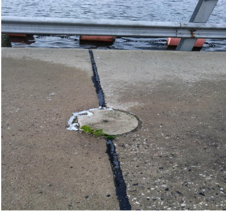
Fig.89: Collecting point of drainage in the main dam body
