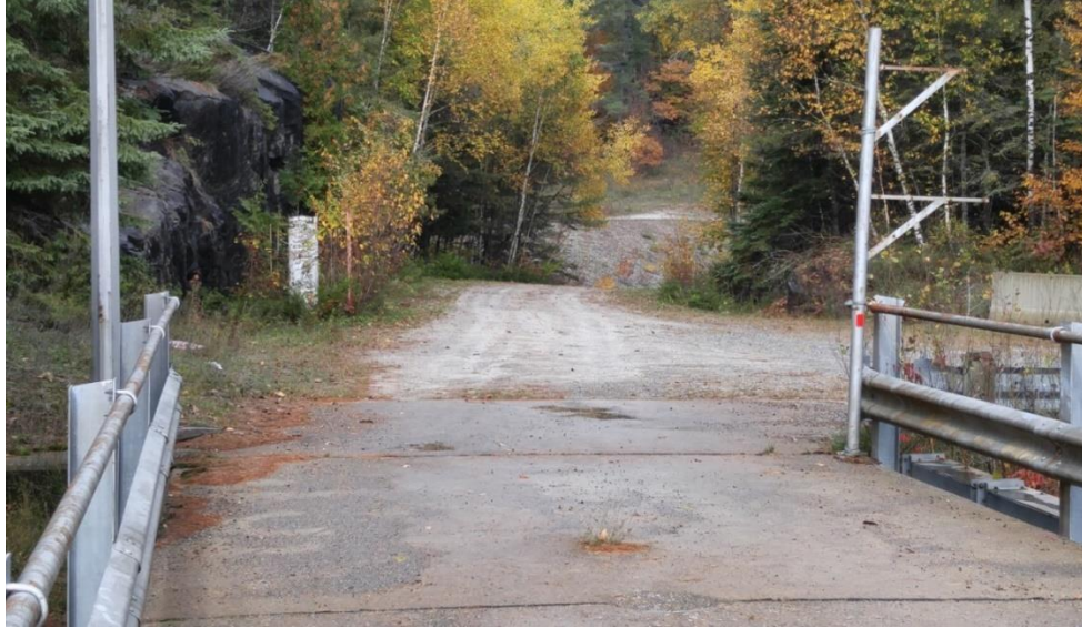
Fig.91: One of the earthen block dams (behind the trees)
