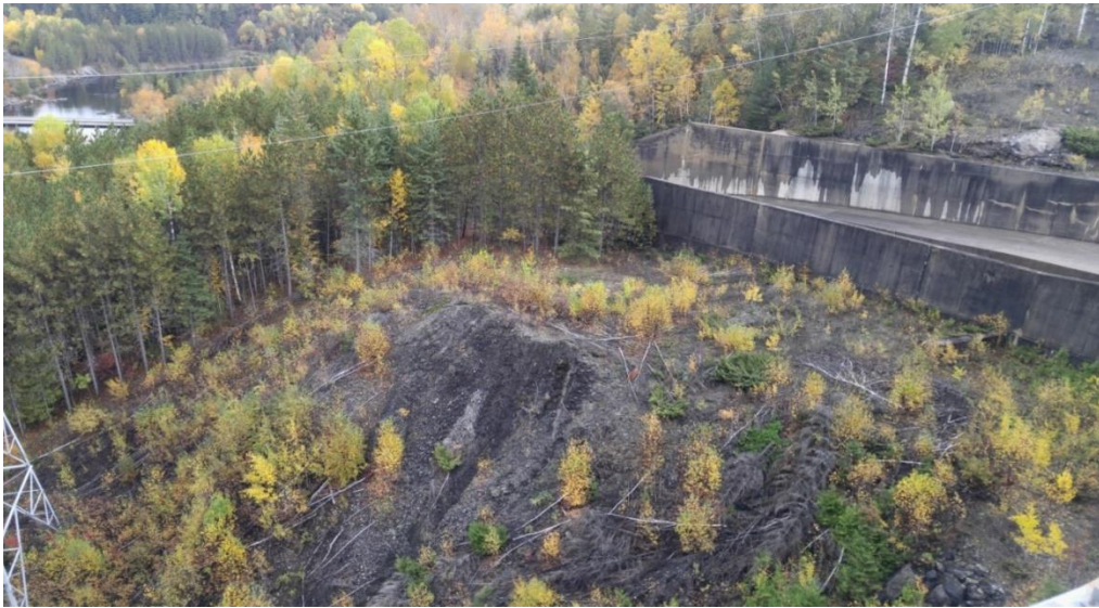
Fig.90: Controlled vegetation around the main concrete dam
