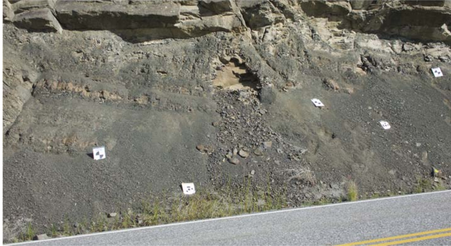
Figure 4 - Example of survey targets placed on the slope
