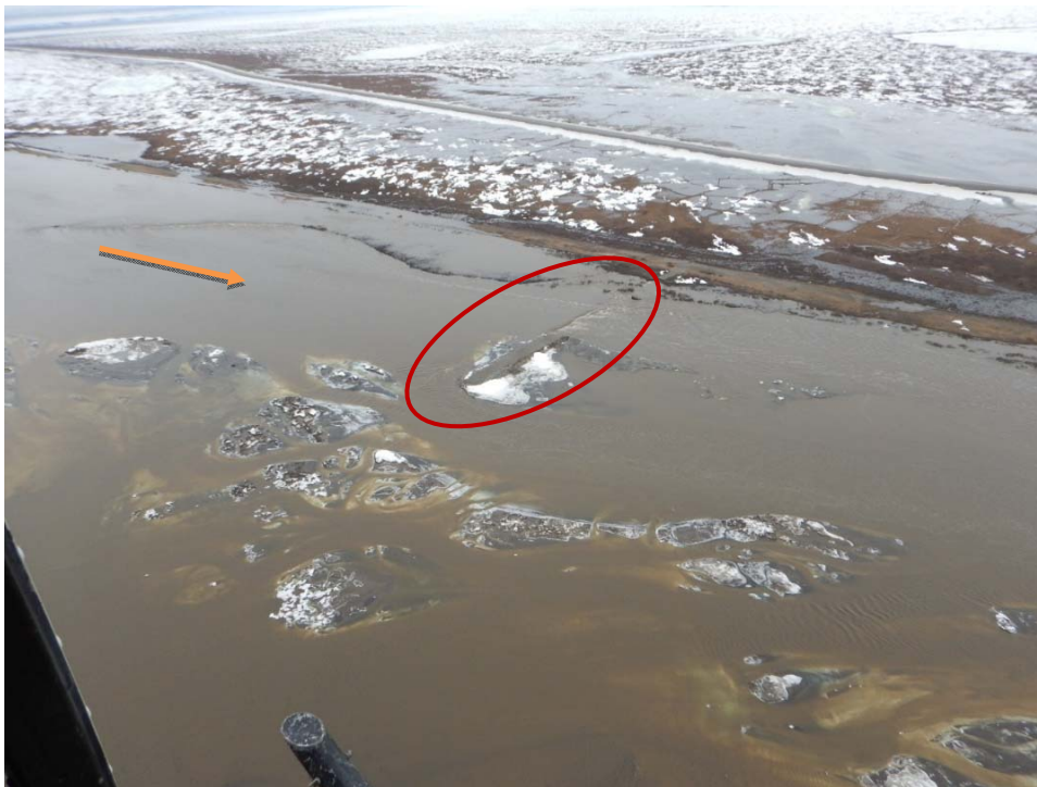
Figure 126. Spur Dike 1 partially breached (within oval) on the Sagavanirktok River near Dalton MP396 on May 30, 2017, during spring breakup. The water is increasingly turbid at the end of spring breakup.
