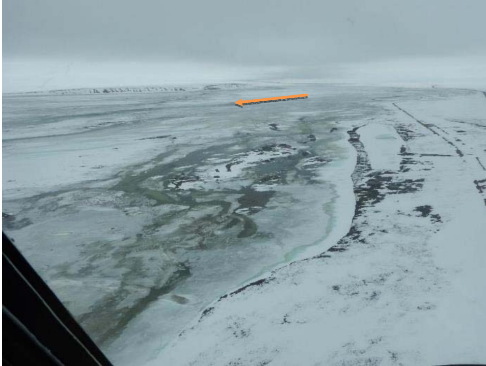
Figure 61. This south-facing view shows the Sagavanirktok River near Franklin Bluffs (visible in left background) on May 20, 2017. The buried pipeline and the Dalton Highway are on the right.
