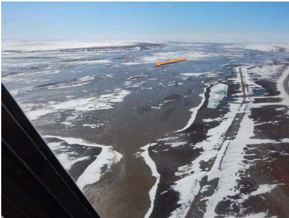
Figure 64. Condition of the Sagavanirktok River on May 27, 2017. Franklin Bluffs appear in the distance; the buried pipeline and the Dalton Highway are on the right. View is to the south.
