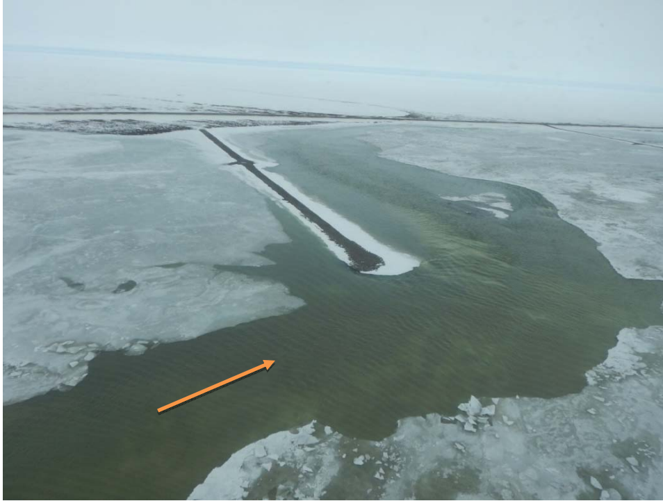
Figure 125. Sagavanirktok River at Spur Dike 2 near Dalton MP396 on May 20, 2017, during early spring breakup. Water is clear and flowing over anchor ice.
