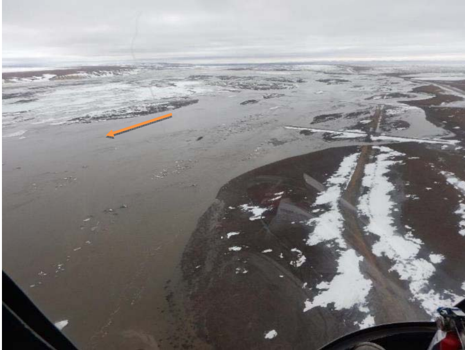
Figure 67. Sagavanirktok River near spur dikes on May 31, 2017 (south view). Franklin Bluffs appear in the distance to the left. The buried pipeline, spur dikes, and Dalton Highway are on the right.
