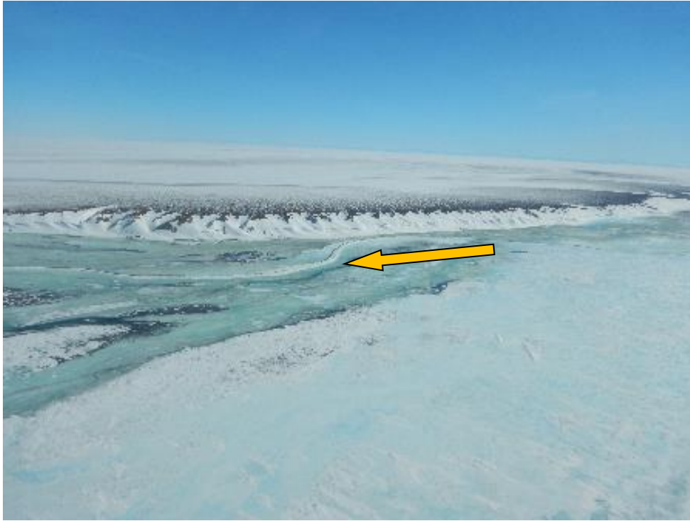
Figure 54. Aufeis on the Sagavanirktok River at Franklin Bluffs and the easternmost trench and berm before significant meltwater inundated the area; view to the southeast. Photo taken on May 10, 2016.
