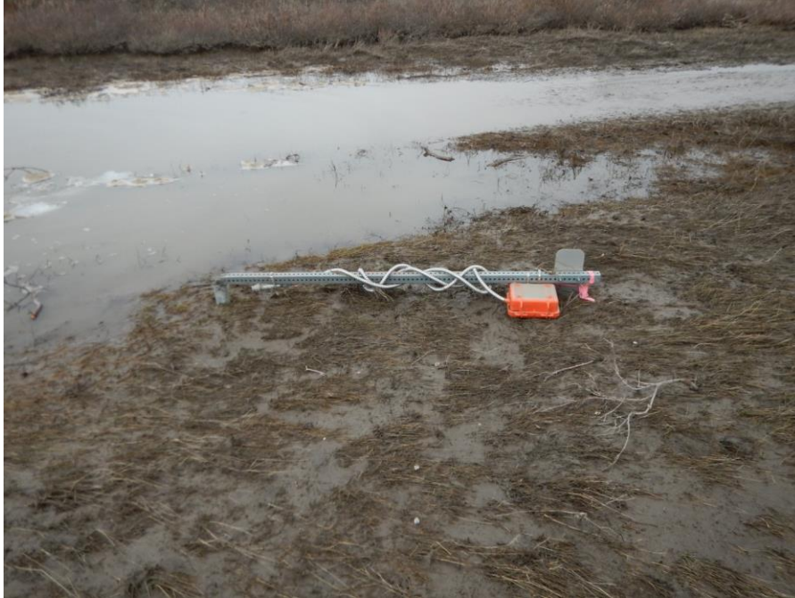
Figure 64. Pressure transducer #10 attached to broken post observed on May 27, 2016.
