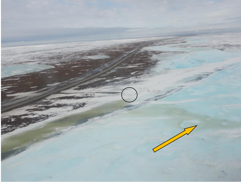
Figure 45. Extensive ice near the west channel of the Sagavanirktok River at MP405 (DSS1) on May 13, 2016. Black circle indicates the station location; view looking north.
