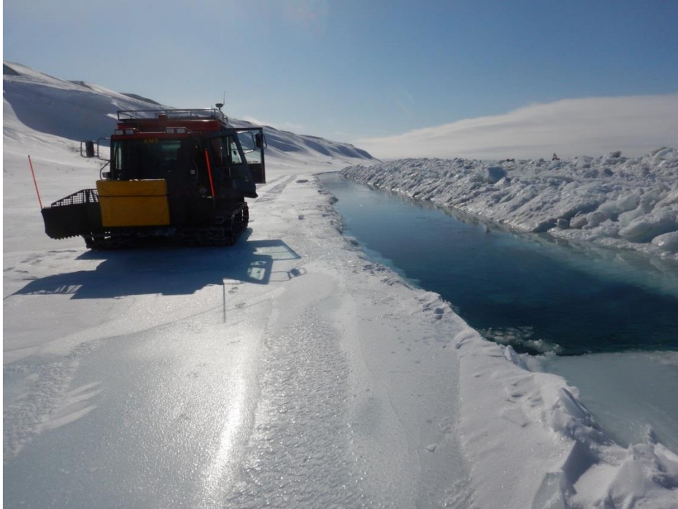
Figure 34. Trench (open water) and ice berm (right side of trench) at Franklin Bluffs on April 17, 2016. The main goal was to improve flow conditions (trench); the secondary goal was to divert initial flow during breakup to the east channel (ice berm).
