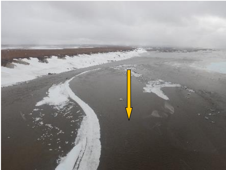
Figure 58. A south-facing view showing the Sagavanirktok River and Franklin Bluffs and the condition of the ice berm at its narrowest point during increased water stage on May 14, 2016.
