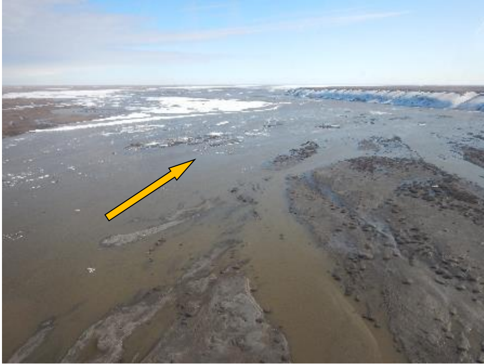
Figure 63. North view showing the still intact southwestern length of the diversion berm on the Sagavanirktok River and Franklin Bluffs on May 27, 2016. Gravel bars are free of ice, and the river is becoming confined to normal channels.
