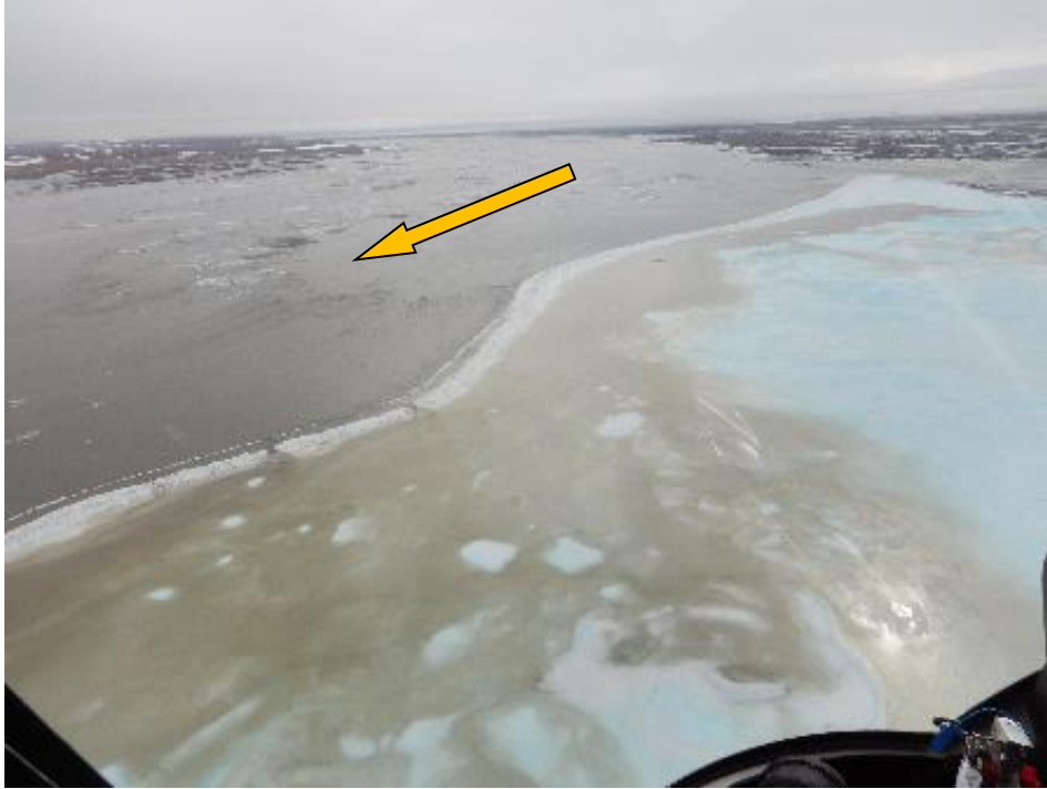
Figure 57. View is south and shows the southwestern length of the ice berm above the narrowing—essentially intact and functioning to divert water to the east during high flow on the Sagavanirktok River near Franklin Bluffs on May 13, 2016. Note in the upper right of the photo that some water has made an “end run” around the southwestern terminus of the berm.
