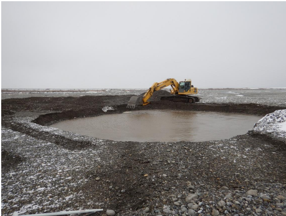
Figure 13. Digging the dry trench at DSS2 on September 10, 2015.
