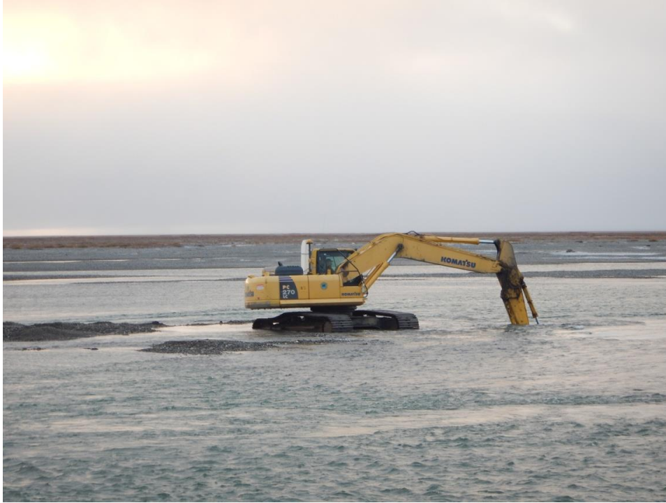
Figure 12. Digging the wet trench at DSS1 on September 9, 2015.
