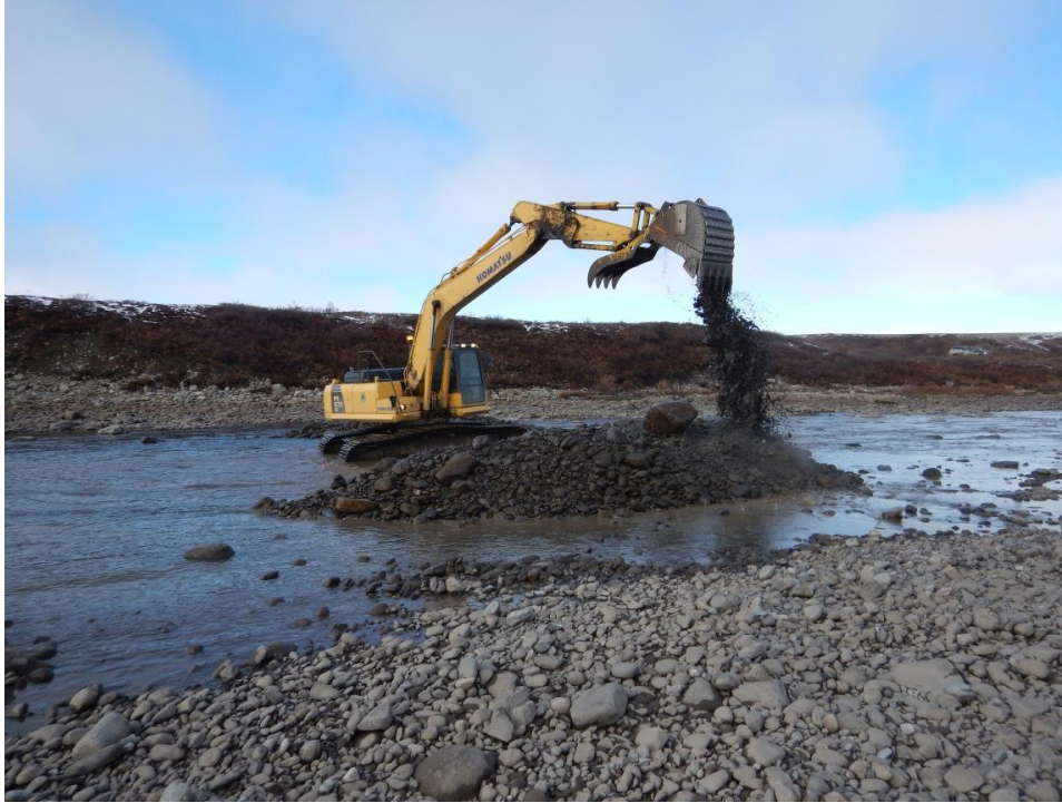
Figure 16. Digging the wet trench at DSS4 on September 15, 2015.
