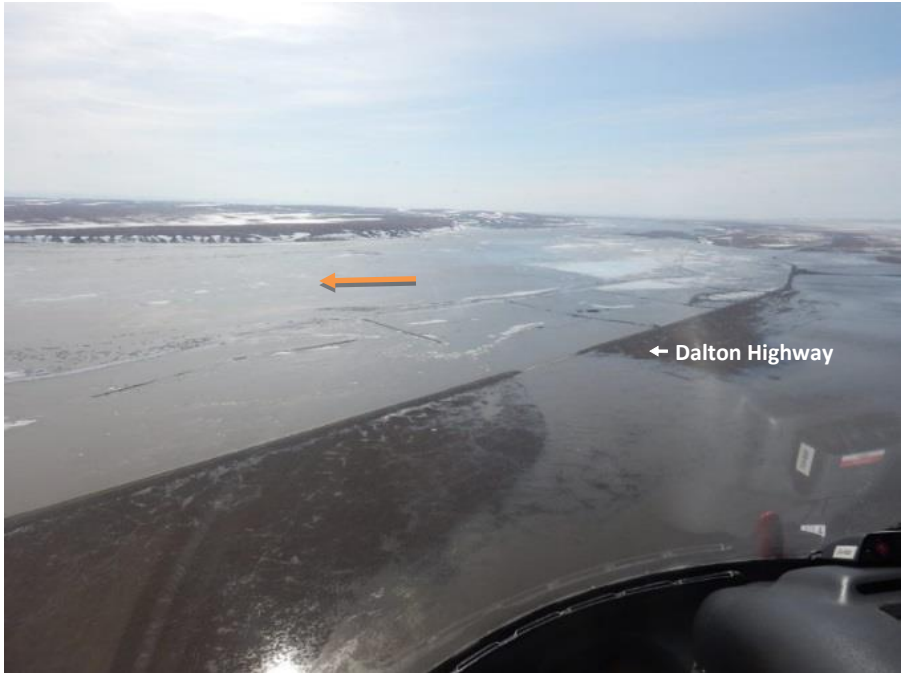
Figure 27. Measurement reach on May 20, 2015, facing southwest, with Franklin Bluffs in the distance. The photograph shows water flowing over the Dalton Highway near the spur dikes. Water levels are very high, and water continues to flow over the ice on the western side of the river.
