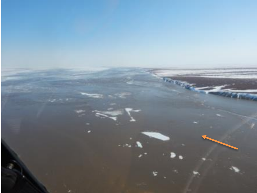
Figure B.23. Photo taken May 18, 2015, near bifurcation of the Sagavanirktok River, View is north. Franklin Bluffs and the diversionary snow dike noted in Figure B.22 can be seen at right. The snow dike is failing, and water covers much of the aufeis seen in Figure B.22.
