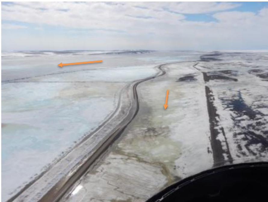
Figure B.4. Photo taken May 17, 2015, near Dalton Highway MP400. View is south and shows the highway on the left and the buried pipeline on the right, converging to intersection. Aufeis is extensive, including area between road and pipeline. Some water is flowing on the ice, and the road is beginning to flood. A Sagavanirktok River channel is at far left, and Franklin Bluffs are seen in the distance, on the horizon.
