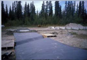
Spanning 12 foot void
