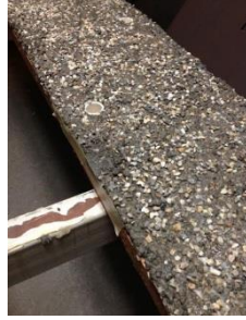
Figure 37: Chip in plank. Figure 38: Chip patched. Figure 39: Additional chip patched.
