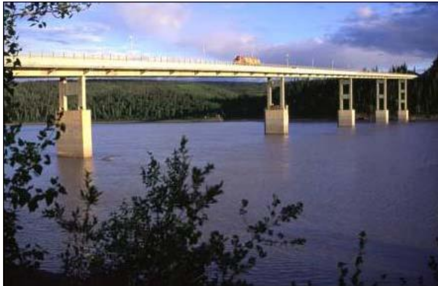
Figure 1: Yukon River Bridge.
