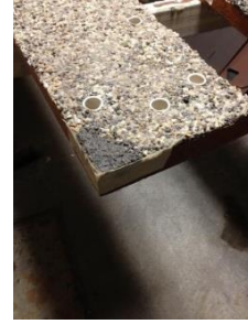
Figure 37: Chip in plank. Figure 38: Chip patched. Figure 39: Additional chip patched.
