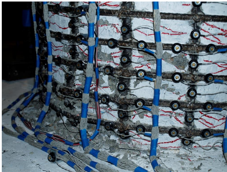
Figure 2.36 Instrumentation Remained Attached to the Latest Stages of Damage
