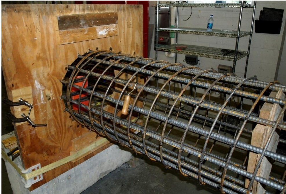
Figure 2.21 External and Internal Column Reinforcement Cage Templates
