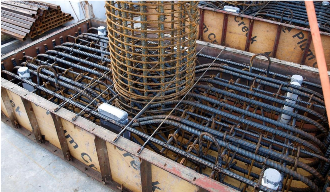
Figure 2.27 Footing Formwork, Reinforcement, Tie Down PVC, and Axial Blockouts
