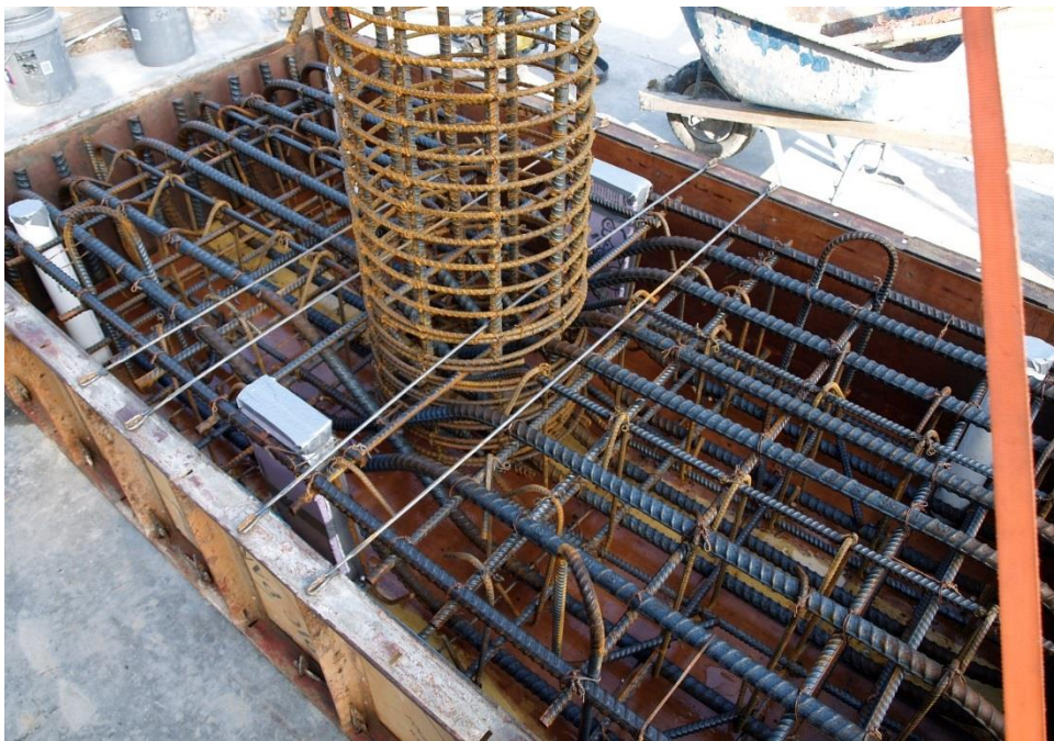
Figure 2.28 Footing Formwork, Reinforcement, Tie Down PVC, and Axial Blockouts
