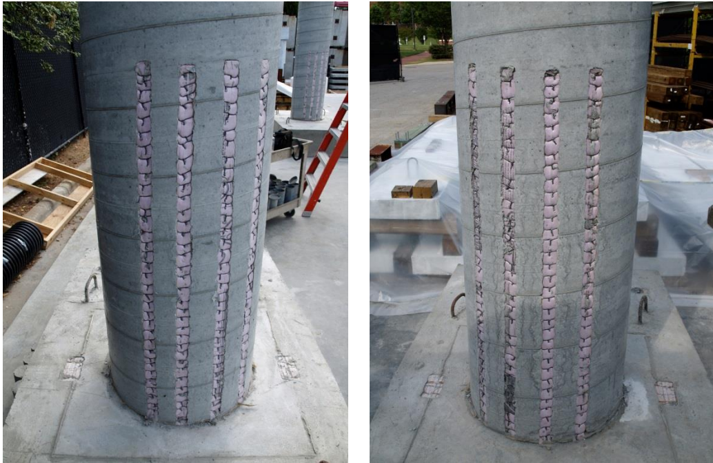
Figure 2.31 After Casting, 2-Layer Longitudinal Cover Concrete Blockout Strips
