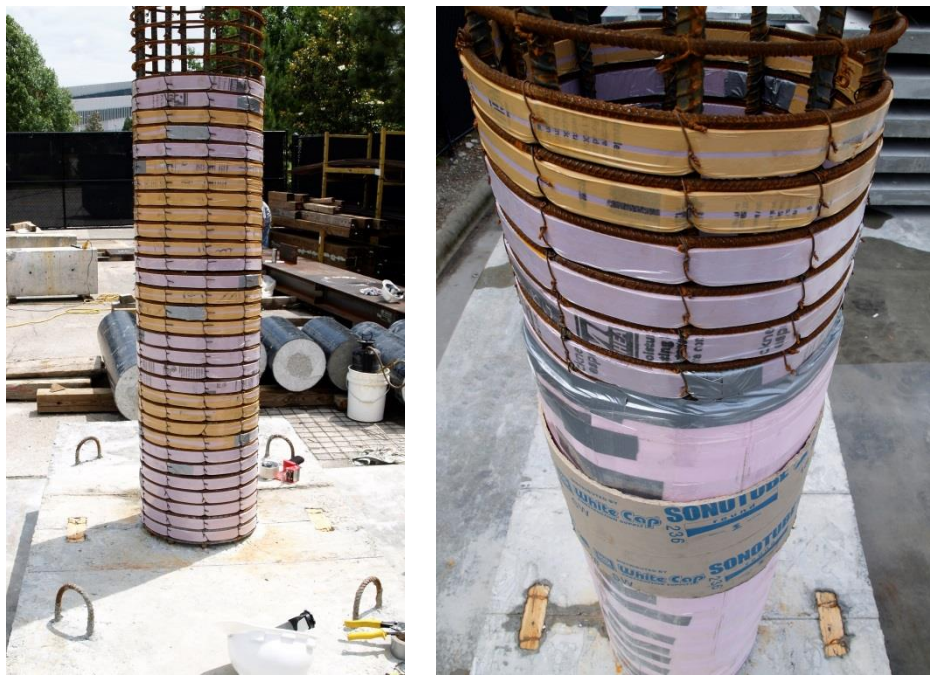
Figure 2.30 Installation of 2-Layer Full Cover Concrete Blockout
