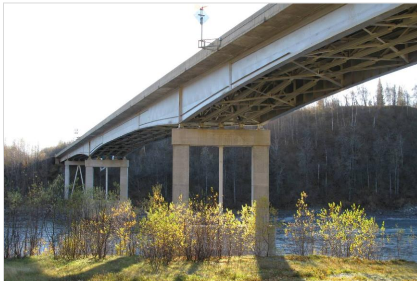
Figure 1.1 Chulitna River Bridge, after 1993 upgrades
