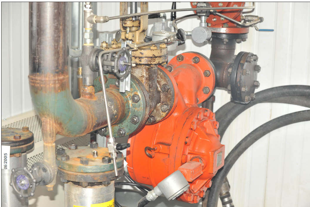
Figure 11. Mixing point for lubricity additive. Lubricity additive enters the fuel stream from the electronic metering system through the smaller gray isolation valve left of center above the large green elbow. The additive mixes with fuel flowing in the larger pipe with a green elbow. The fuel and the additive mixing is assured as the components flow through the meter (orange) and on to the awaiting truck. Photo by Frank Williams.
