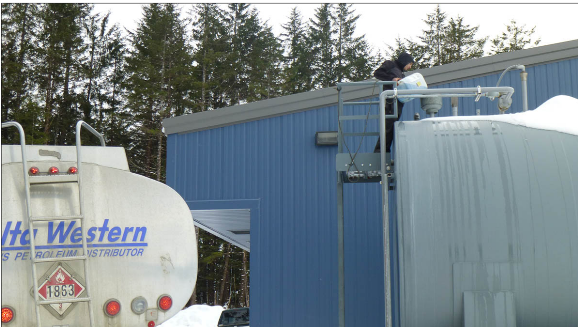
Figure 13. "Splash blending" of an additive at the Yakutat Power for testing purposes. Note fuel truck delivering fuel to the power plant and the worker adding a liquid to the tank during fuel delivery, using the mixing provided by the fuel movement during transfer to mix the additive with the fuel. Photo by Scott Newlun.
