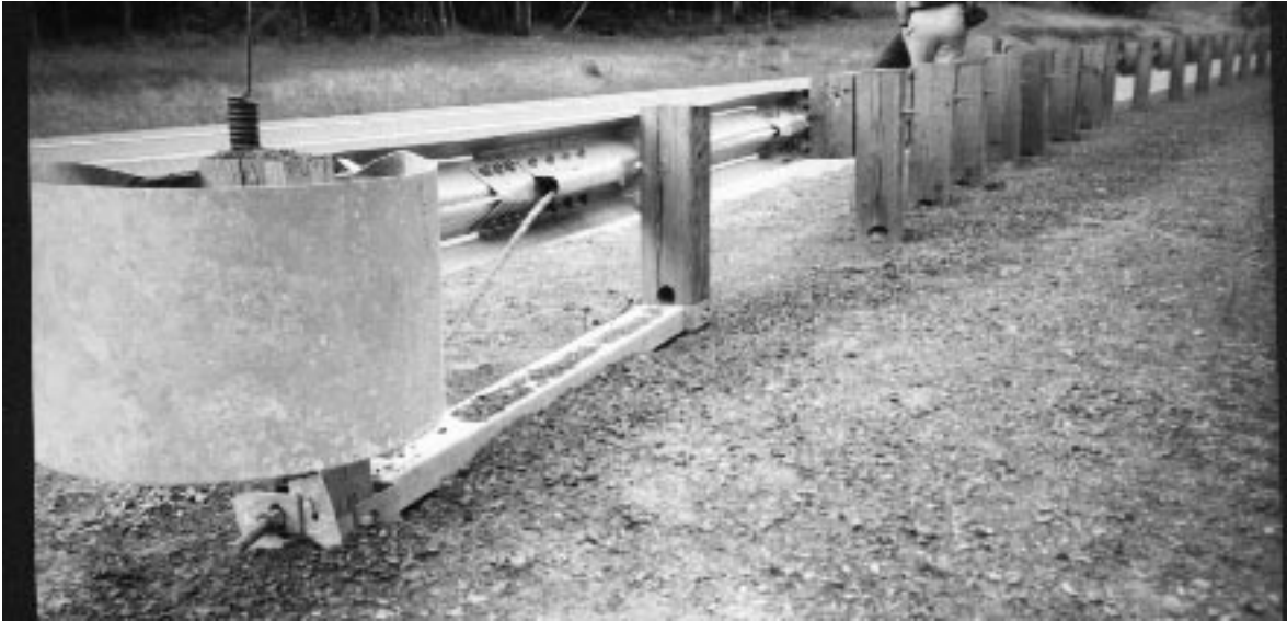
Fig. 2 Wooden Posts with Holes
