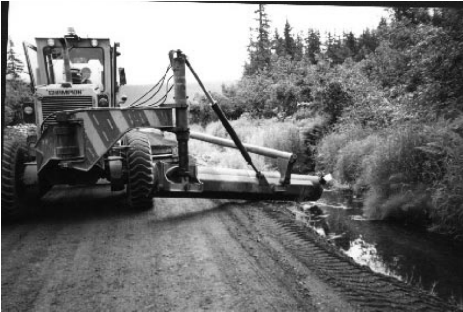
Fig. 4 A Grader with a Sloper Attachment
