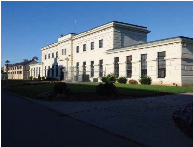
Figure 9: Administration building at Prison 2
