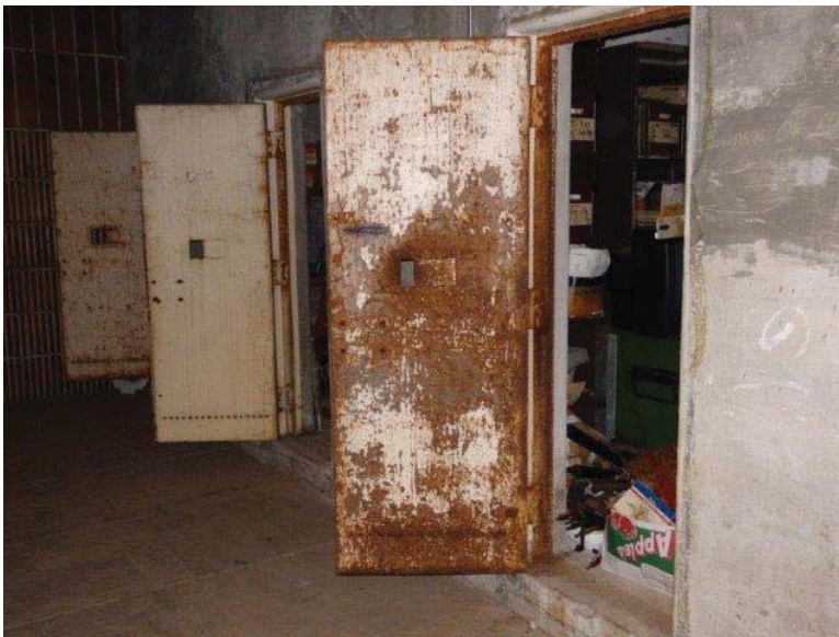
Figure 14: View of original solitary confinement cells in Prison 2
