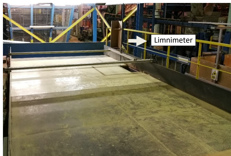
Figure 4:4 Graphics with the structure to support limnimeter.
