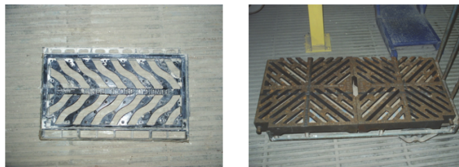
Figure 3:2 Two types of grates ( Types 10 and 11) used to validate the methodology carried out.
