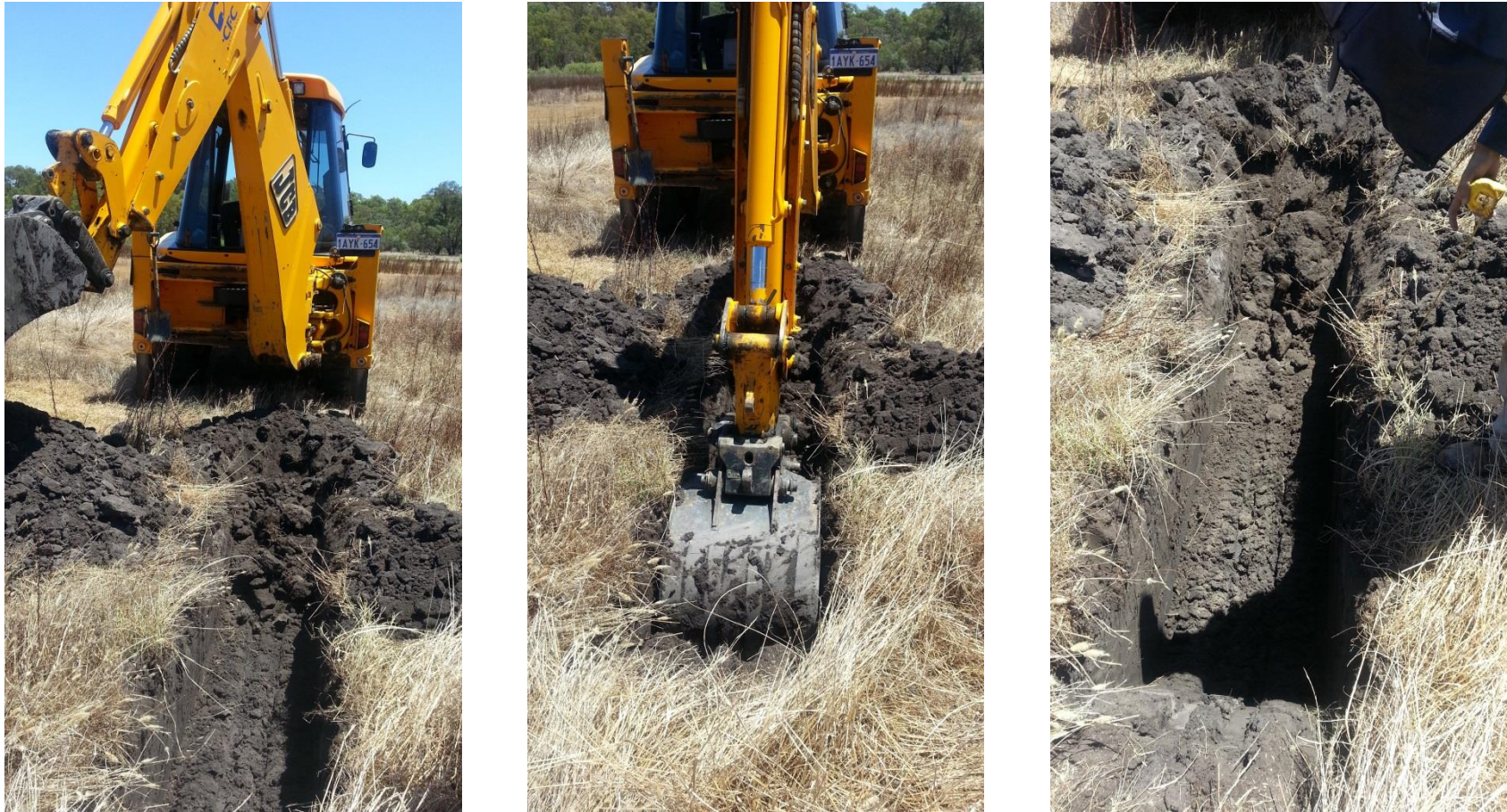
Figure A.1 . Test pitting procedure
