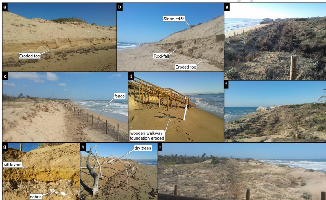
Figure 9: Mosaic with representative images. (a) Dune toe eroded in zone 3. (b) Slope of the artificial dune in zone 1, with the toe eroded and landslides due to regrading. (c) Erosion of the dune, the fence marked the dune toe in 2007. (d) Foundation of the wooden walkway in the air due to erosion. (e) View of vegetation on dune in 2015 and (f) in 2017. Note the loss of vegetation. (g) Layers of silt and debris on the artificial dune in zone 1. (h) Dry trees due to shoreline erosion. (i) View of the state of vegetation on the foredune in zone 2.
