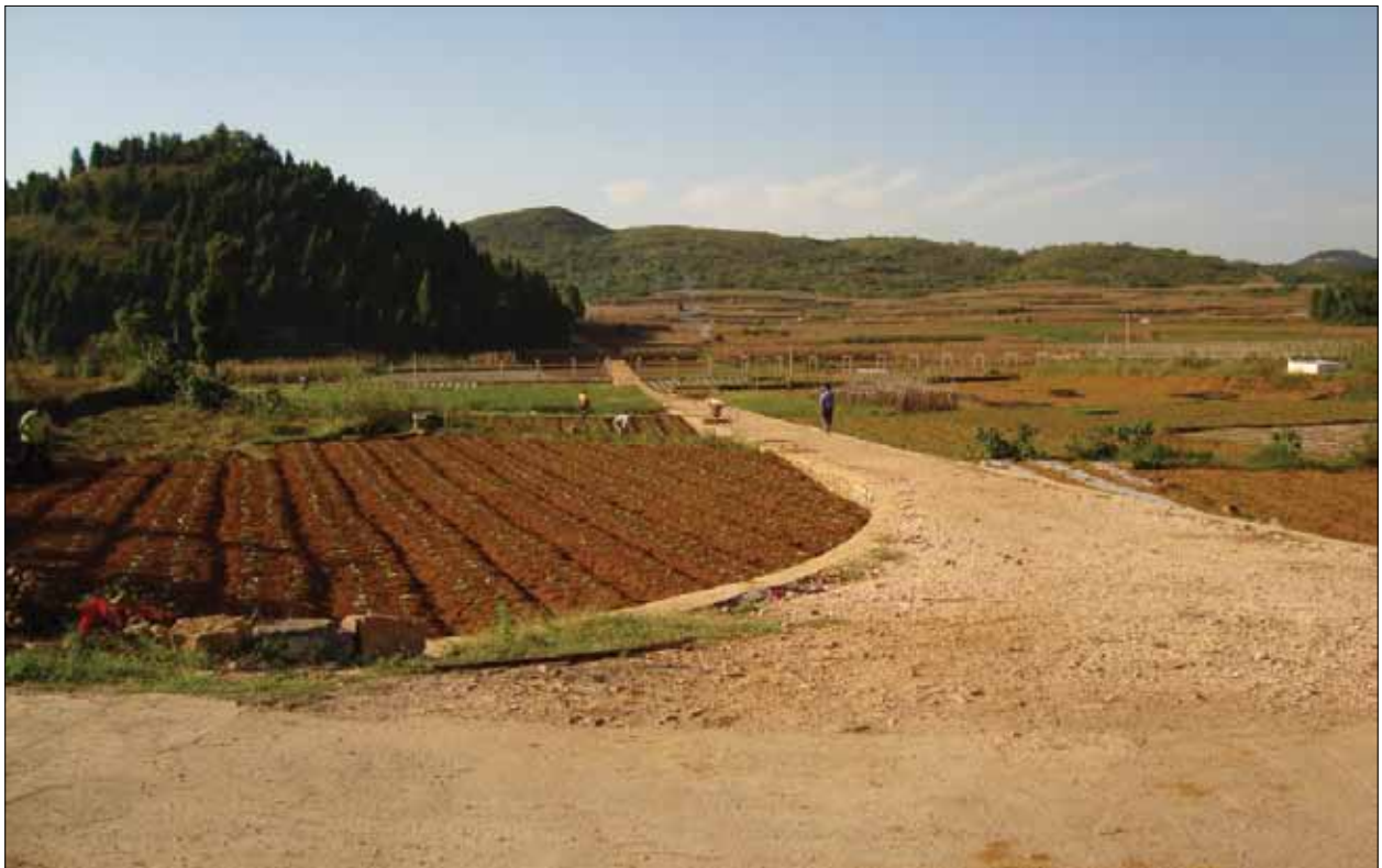
Figure 16 to 17. Village roads constructed from project support with collective action.
