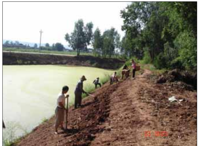
Water harvesting structure
