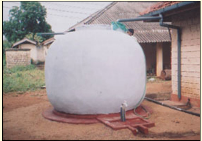
Domestic rainwater harvesting tank, Sri Lanka.
