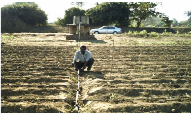
Fig. 1 Front view showing drip main line from the drip tank raised 1.5 m on concrete
