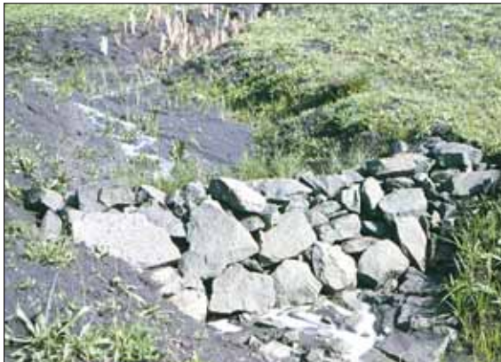
Figure 9. Loose rock check-dam for gully control in Ginchi watershed, Ethiopia.
