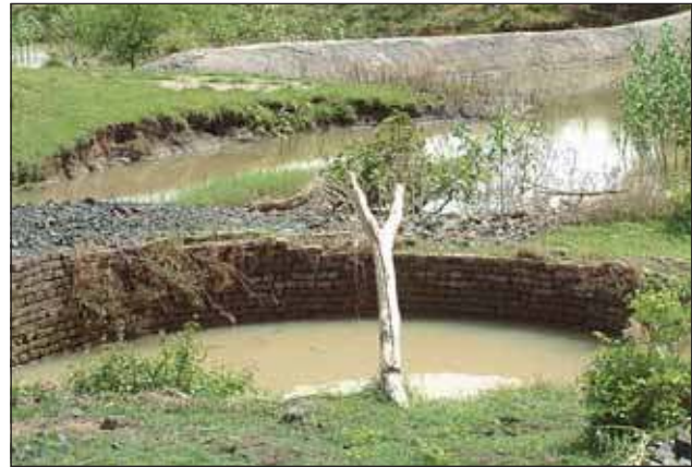
Figure 26. A recharged well near a gully control structure in Mudhsudhangadh watershed, Madhya Pradesh, India.
