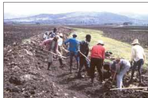
Figure 6. Farmers making diversion channel for controlling gully erosion in Ginchi watershed, Ethiopia.
