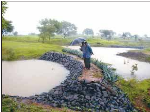
Figure 21. Mini-percolation tank for recharging groundwater and controlling gully erosion in Kothapally watershed, Andhra Pradesh, India.
