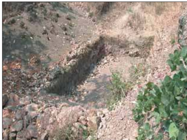
Figure 22. Sunken pits in the gully bed at Kothapally watershed, Andhra Pradesh, India.
