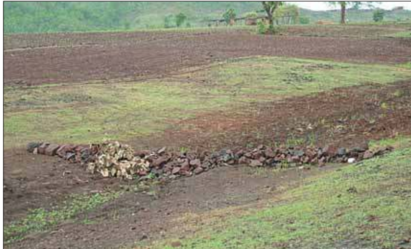
Figure 5. Control of a small gully through small stone structure.
