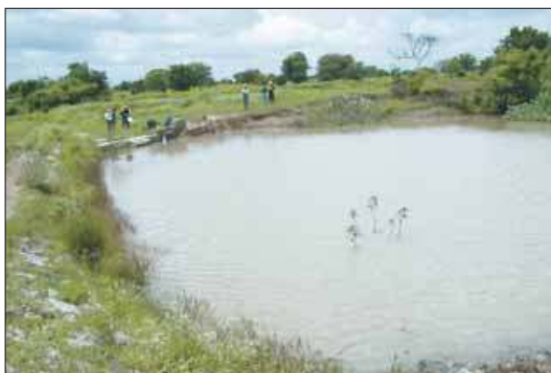
Figure 24. Earthen check-dam with outlet in Kothapally watershed, Andhra Pradesh, India.
