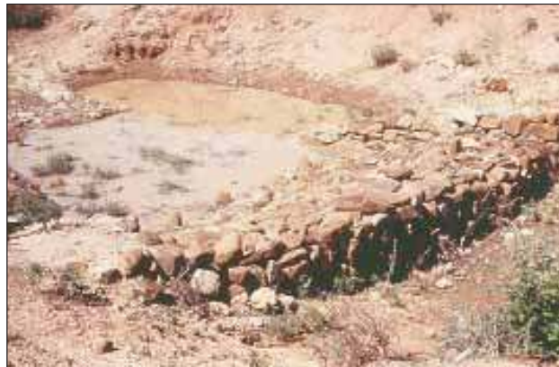
Figure 10. Loose rock drop structure for controlling gully erosion in Mittimari watershed, Karnataka, India.
