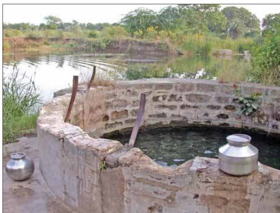
Figure 10. Open well water level is up to the ground level recharged by water harvesting structure (WHS).
