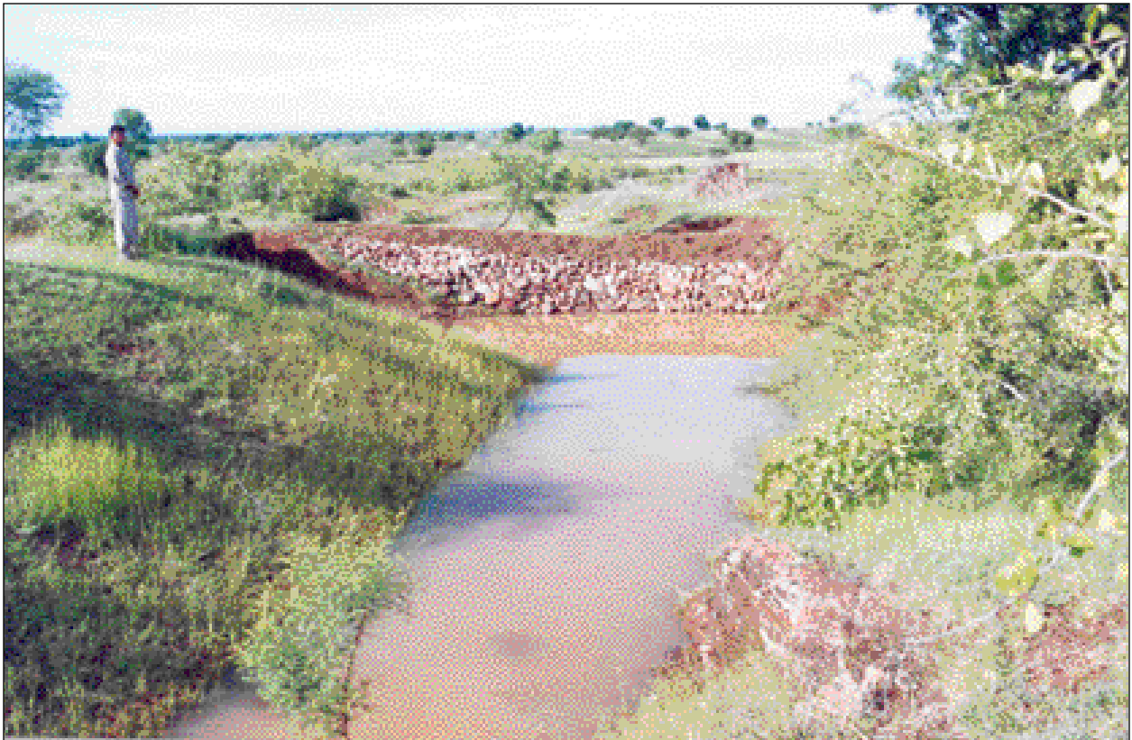
Figure 8. Low-cost mini-percolation structure for groundwater recharging.
