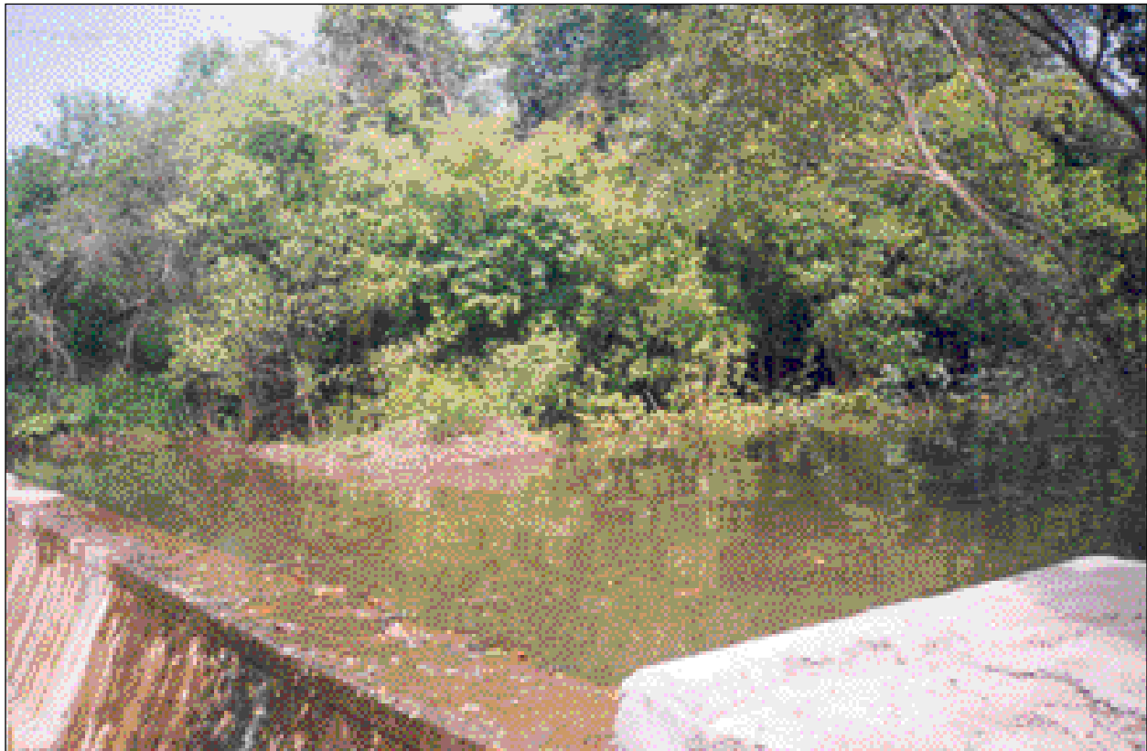
Figure 6. Check dam conserving runoff water in the village.
