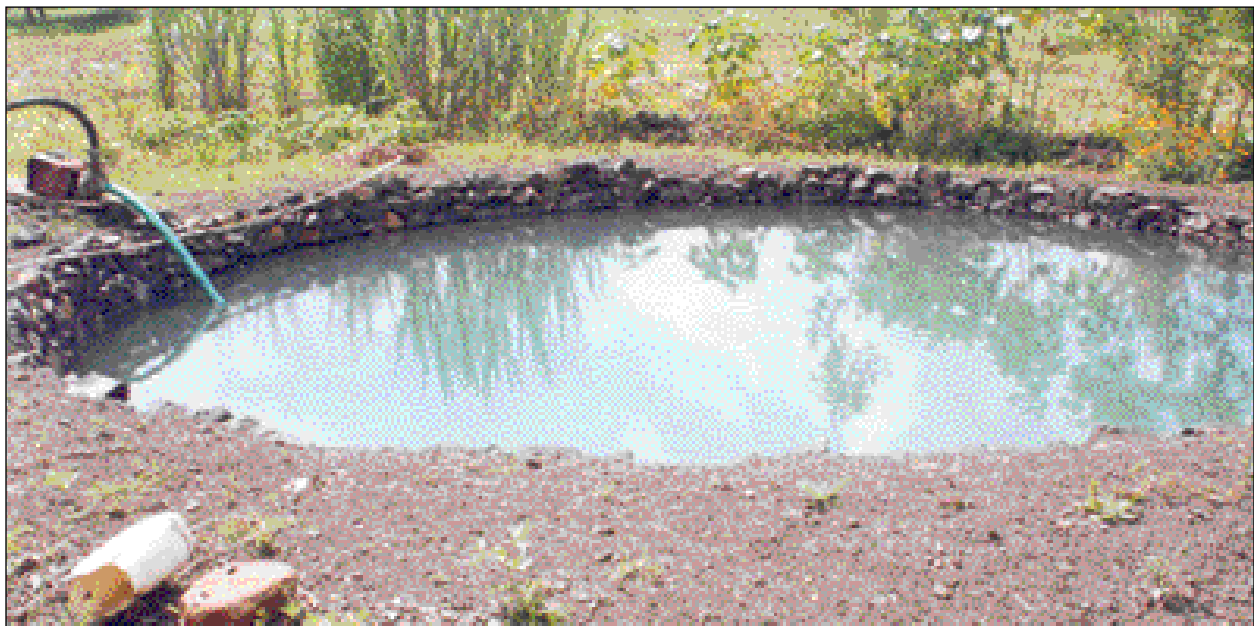
Figure 11. A recharged well with pump for irrigation.
