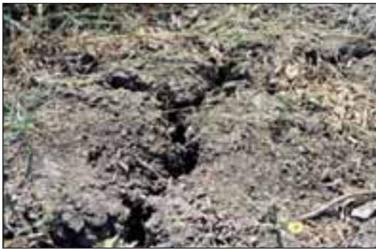
Wide polygonal cracks at the benchmark spot
