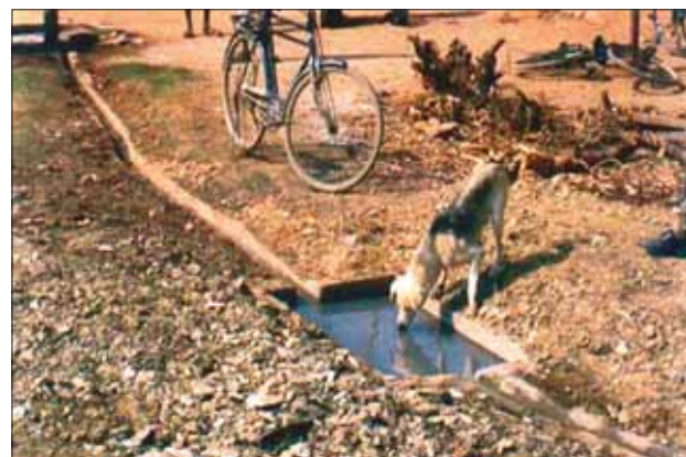
Figure 22. Soak pit constructed at Gokulpura village.
