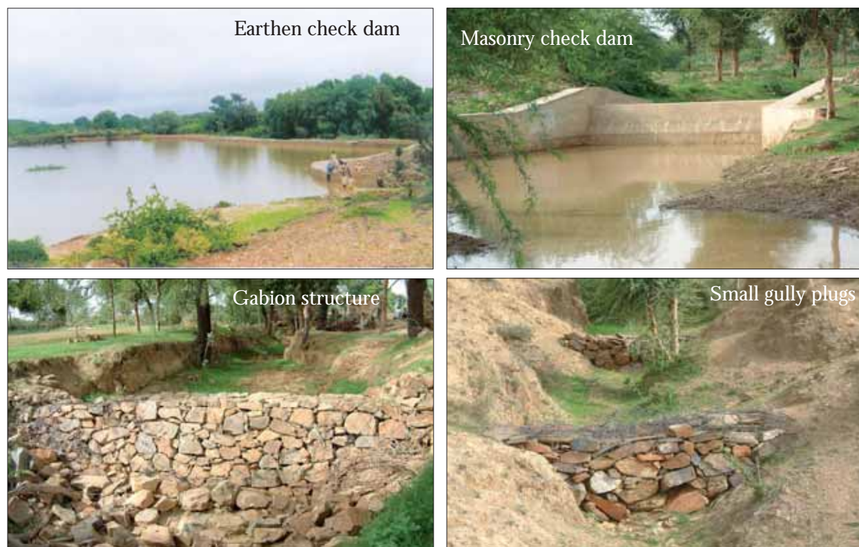
Figure 8. Various soil and water conservation structures at Gokulpura-Goverdhanpura watershed.
