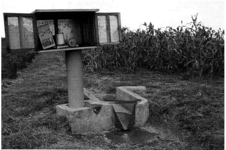
Figure 4 — H-flume attached to a stilling well and connected to a drum-type recorder for measuring runoff.
