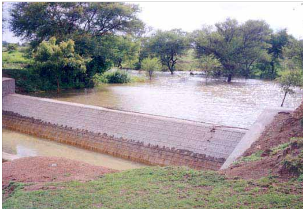
Figure 4. Water stored in check dam built across the stream channel (ex-situ management); Photo: Kothapally watershed.
