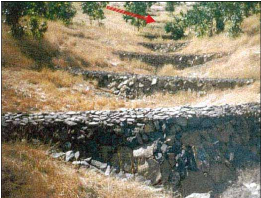
Figure 14. Series of loose boulder wall gully checks at Bundi watershed, Rajasthan.
