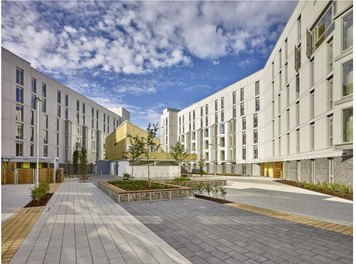
Figure 3.2 Architectural design image made LSI Architects. Left, Barton House, Central building and Right Hickling House
