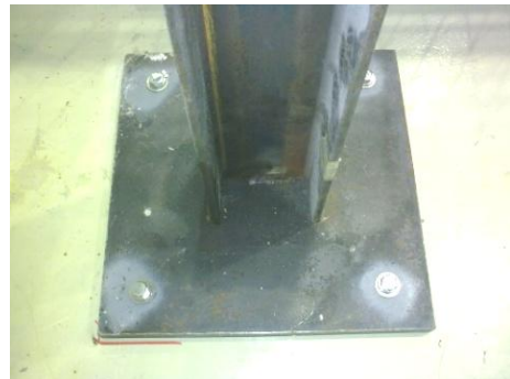
(f) Column-base connection on the right
