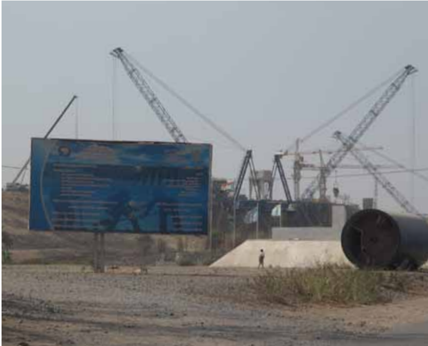
784, 782, 783.jpg: Construction work on the dam.
