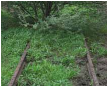
616.jpg: The overgrown railway line
