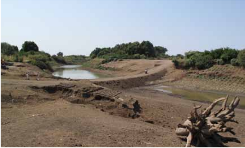
934jpg: The crossing of the Rahad river between At-Tayba and Baazuura. Of the water only standing pools are left. The dam for the road obviously must be rebuilt every year after the flood.
