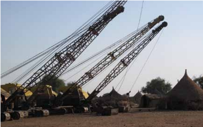
679.jpg: Machines for the excavation of the new canal.
