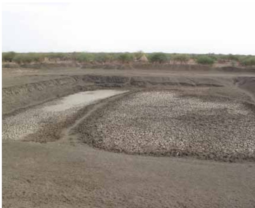
659.jpg: The hafir , the water reservoir dug for run-off surface water in the wet season, has dried up three to four months earlier than last year. (PHOTOS: G. SCHLEE)
