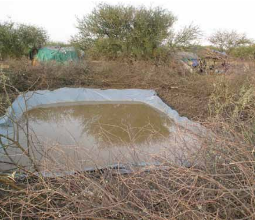
664.jpg: Some of the water which is brought by lorry and bought for four SDG per barrel is poured into this plastic-lined 'small hafir '. Losses by evaporation must be high. Adam has also hired a tank of the type used on lorries to keep water for his smallstock. There are no losses by evaporation there, but the rent of the tank is 80 SDG per month. (PHOTO: G. SCHLEE)
