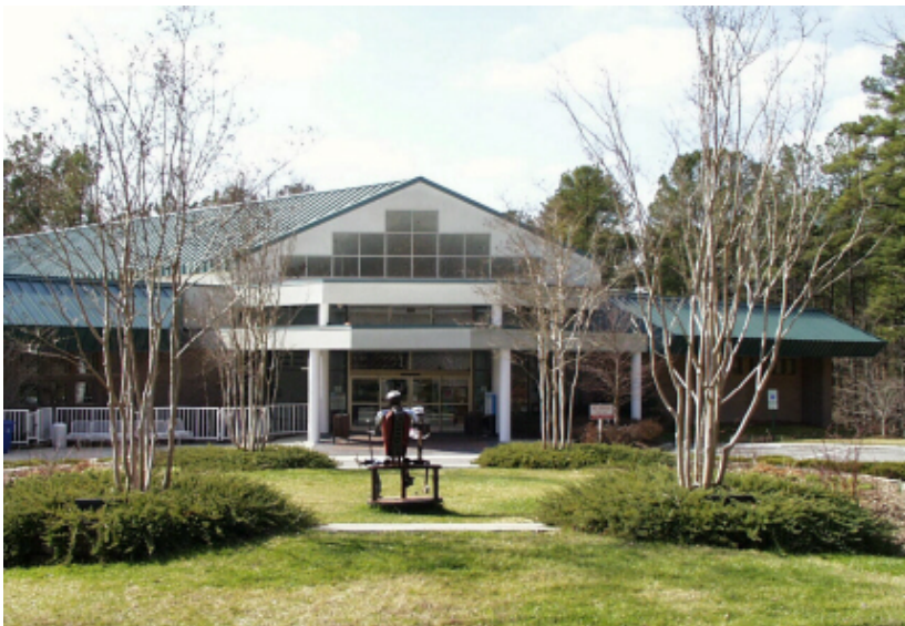
Figure 2: Exterior of library before renovations (GGA Architects)
