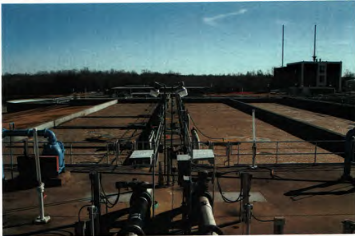
Photograph 1. IFAS (left) and ASP (right) during testing (January). Photograph taken by the author.
