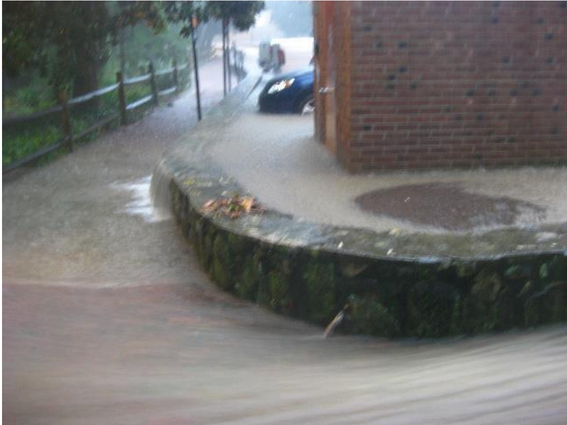
Figure 7: Surcharging of Inlet 221 Adjacent to Pump House (MacIntyre) (Note overtopping of wall, and water level around car tire in top center of photo)
