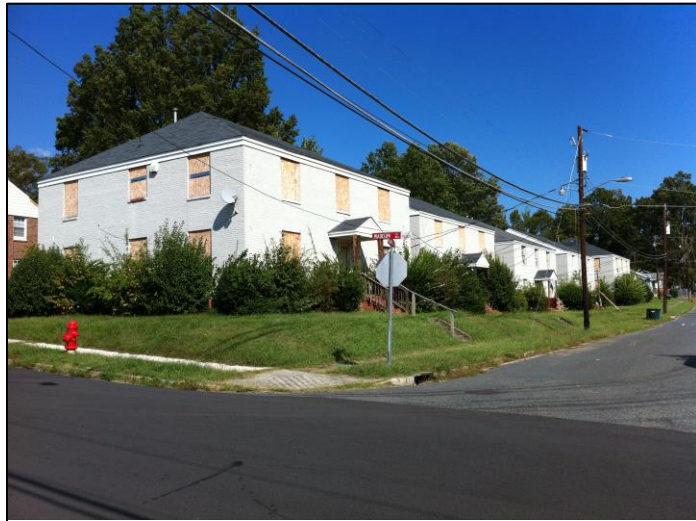
Figure 4 - North Street Before Renovations
