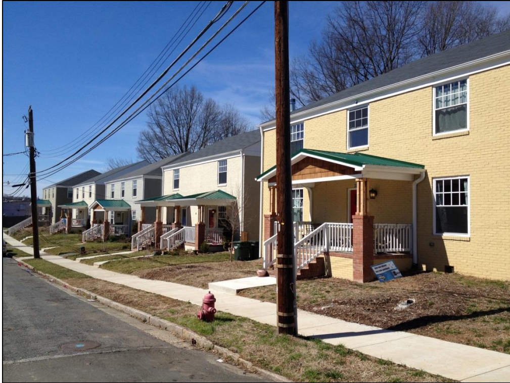
Units completed along Northwood Circle
