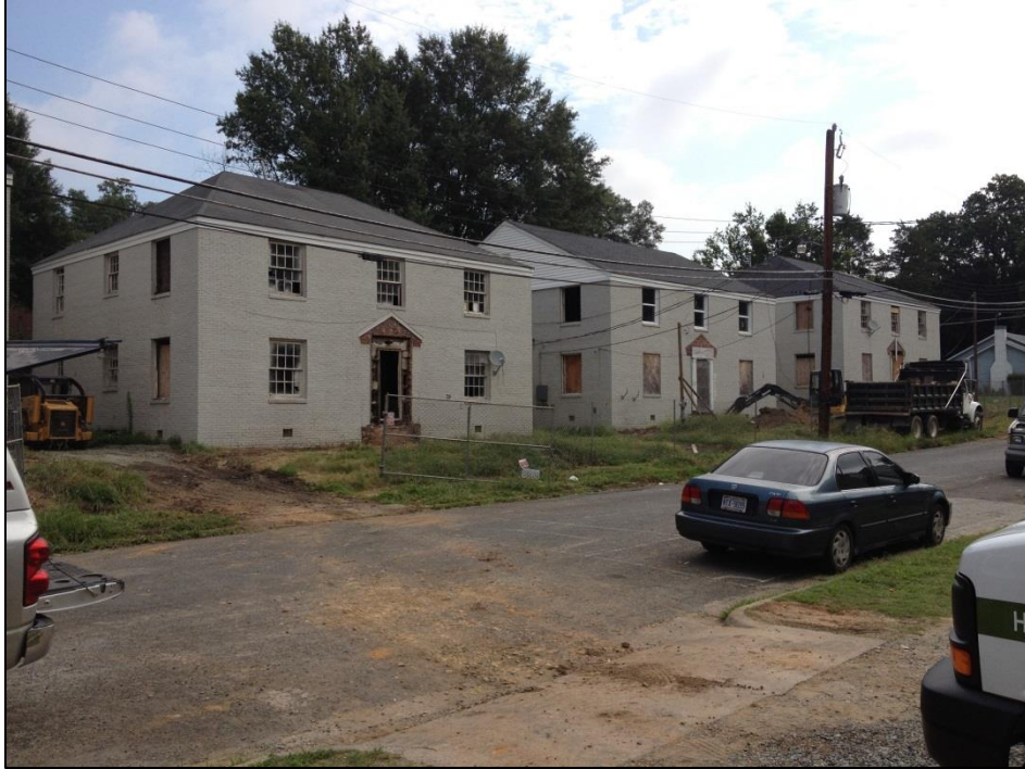
Start of the redevelopment on Northwood Circle
