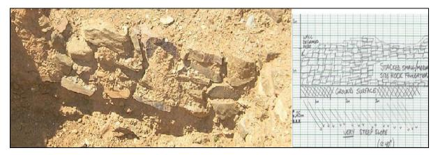
Figure 4-10. Stacked stone masonry wall, photo with field map in profile
