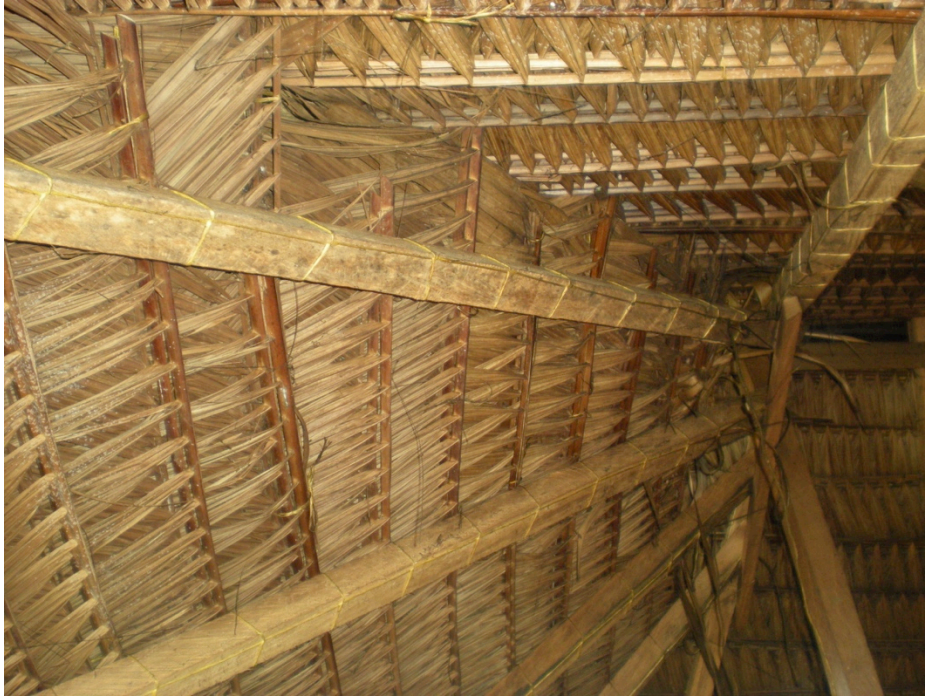
Figure 84. Touring a Self-Sufficient Farm #1: An alter-roof for an alter-politics. The house's locally-harvested and built thatch roof. Source: Author photo.
