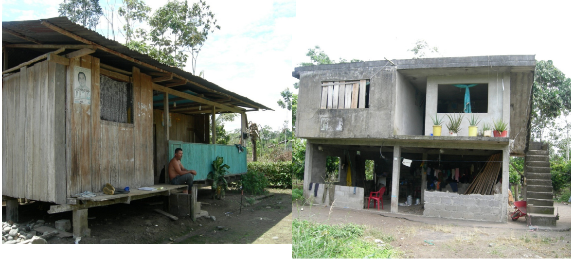
Figure 4.1. House types existing in the study area. Left wood house type, right cement house type. Fieldwork, summer 2007, P. Polo.
