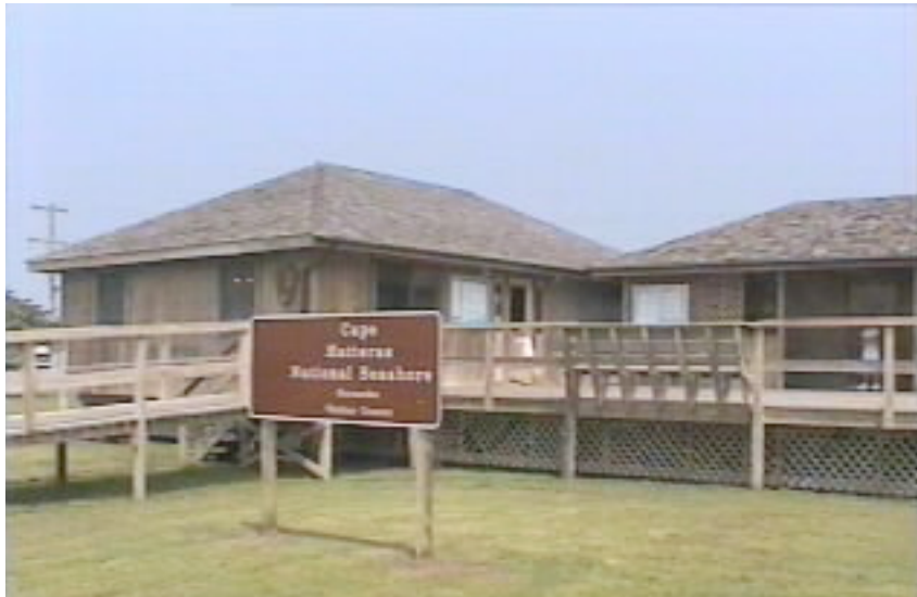
Figure 4.5: Exterior front view of the Ocracoke Visitor Center
