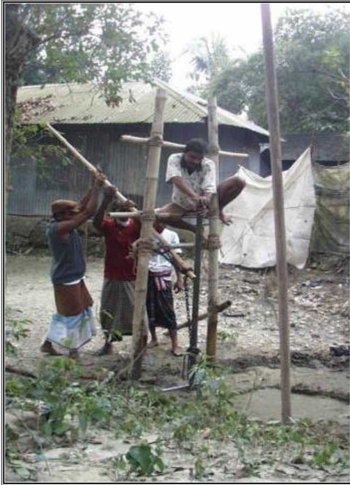
Figure 1.1: Tubewell installation
