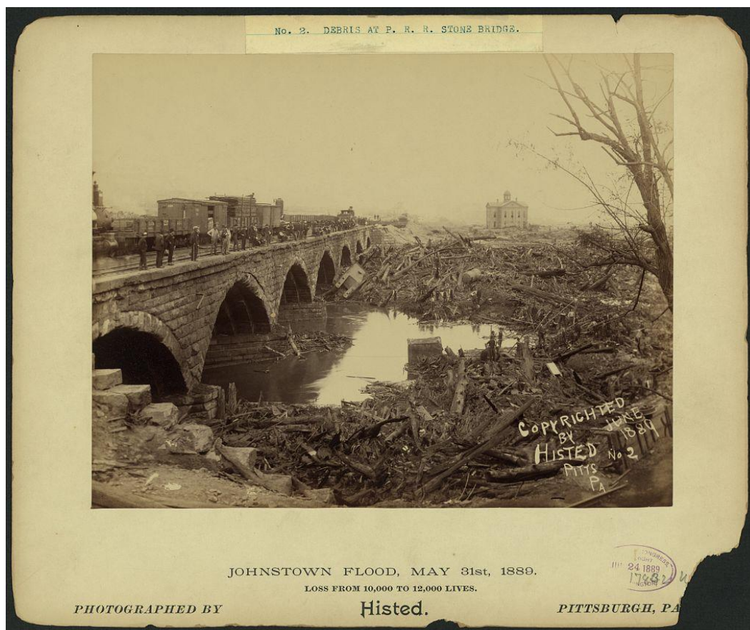
Figure 7. Ernest W. Histed, Debris at P.R.R. Stone Bridge , 1889. http://www.loc.gov/pictures/item/2002707085
