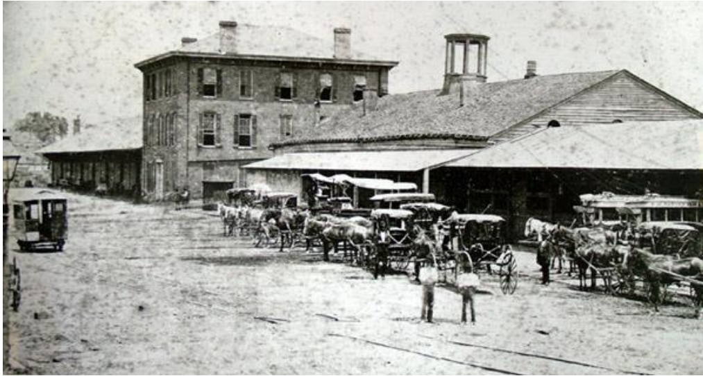
Figure 29. Memphis and Charleston Depot, ca.1880.
