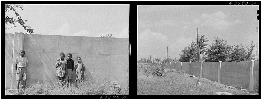
FIGURE 1. Detroit Wailing Wall in 1940s (Source: Library of Congress).
