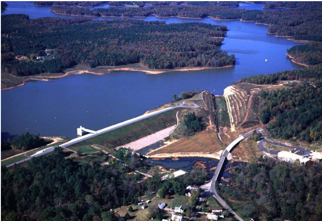
Figure 19: Falls Lake Dam on Falls Lake near Raleigh. Photo copyright of the US Core of Engineers
