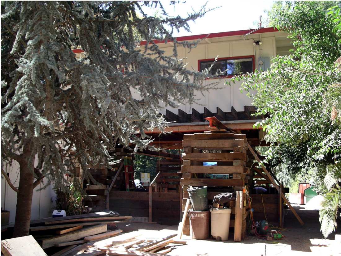
Figure 47: Felton Grove elevation project in progress. Photo by Danny de Vries 2004.
