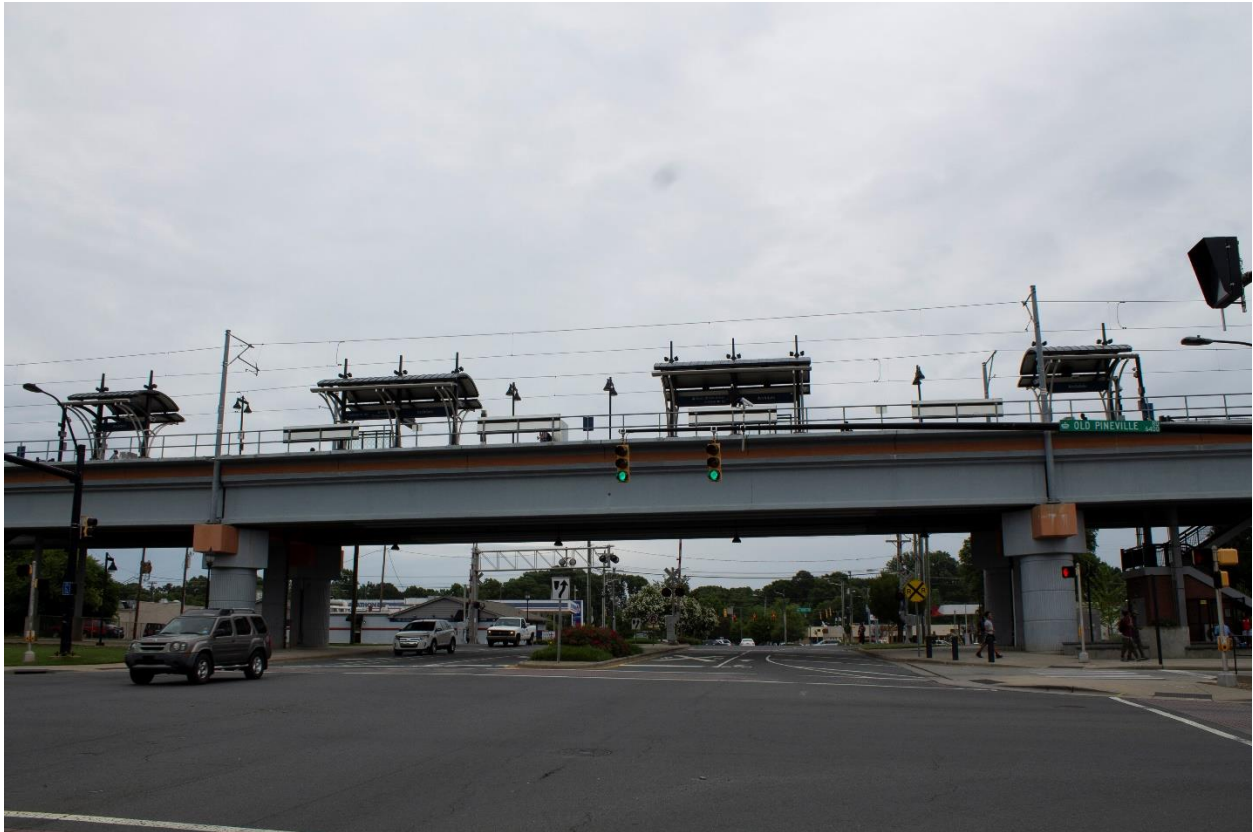
Figure 4.19 Looking at Archdale Drive towards South Boulevard. Signalized crosswalks, a bike lane on Archdale Drive, and a median are attempts to make this space more pedestrian friendly.
