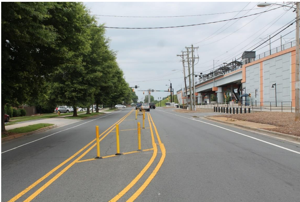
Figure 4.20. Old Pineville Road.
