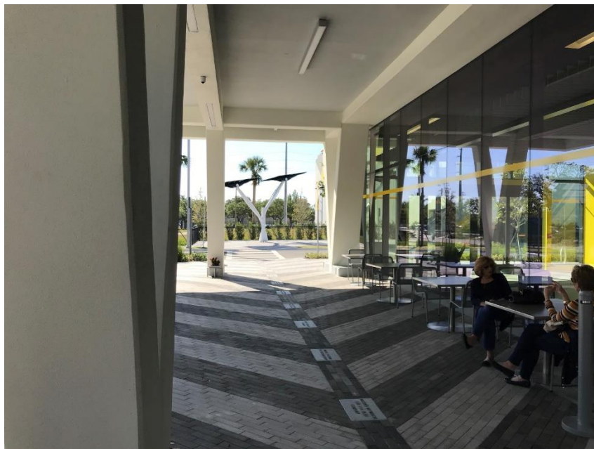
Figure 5.3. This is a photo of the private pedestrian experience at the Fort Lauderdale Brightline station. Comfortable seats and tables, shaded, well-lit entrance to the station. Modern amenities such as solar panels and pavers. A sense of security. Separation from cars.
