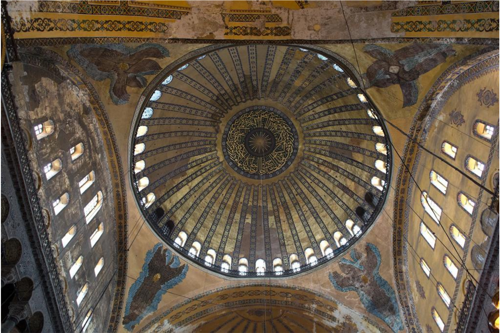
Dome with four seraphim painted on the pendentives, Hagia Sophia, Istanbul, Turkey, Isidore of Miletus and Anthemius of Tralles, 532-537
