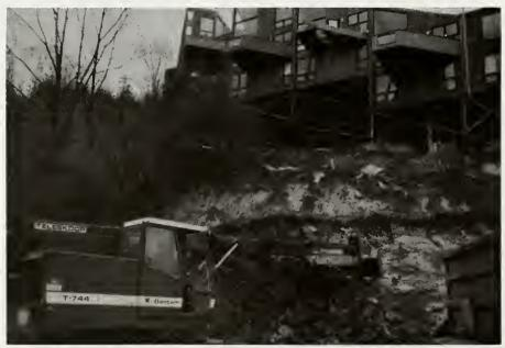
Extensive grading of hillsides makes them susceptible to landslides and erosion.
