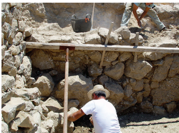
Figure 2. East wall of the Communal Dining Building, temporarily stabilized during conservation (Photo: Azoria Project)
