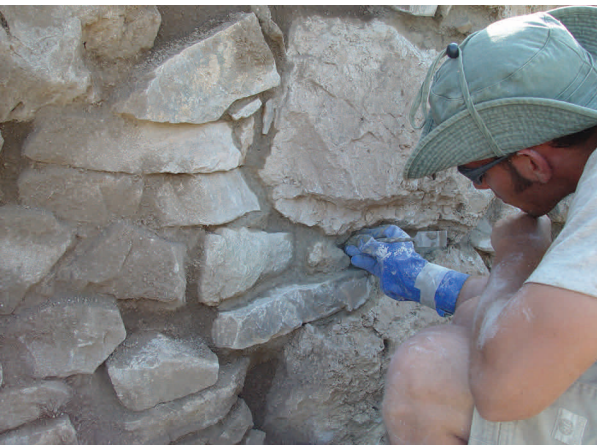
Figure 10. Scraping and cleaning applied mortar (Photo: Azoria Project)
