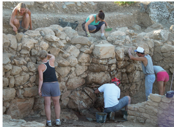
Figure 5. Using hand tools to remove the earth mortar (Photo: Azoria Project)
