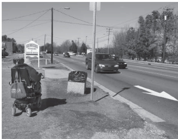
Example of bus stop deficiencies: Lack of level lift areas can be an issue for wheelchair users at bus stops. Image courtesy of authors.
